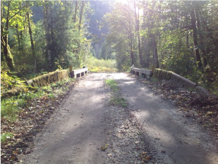
Approach from Right Bank when facing downstream
