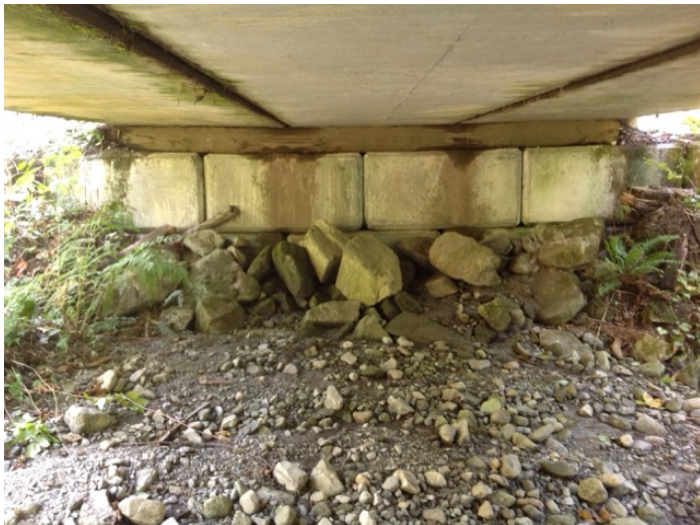
Left Bank Abutment when facing downstream
