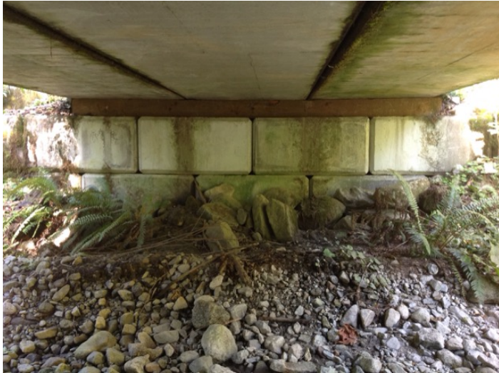
Right Bank Abutment when facing downstream
